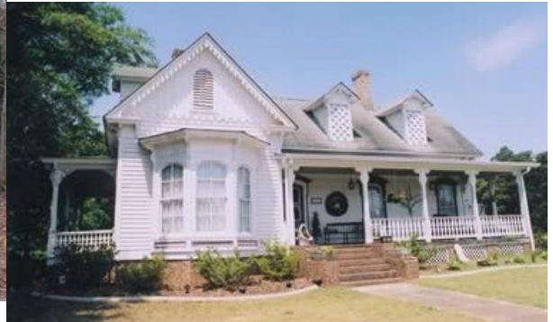
Richard White House: C1900's ready for re-construction to 3,000sf...
